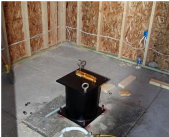
The pier riser was designed to fit on the existing pier anchor. The re-painted pier bolted to the top plate of the riser – easy peasy.
