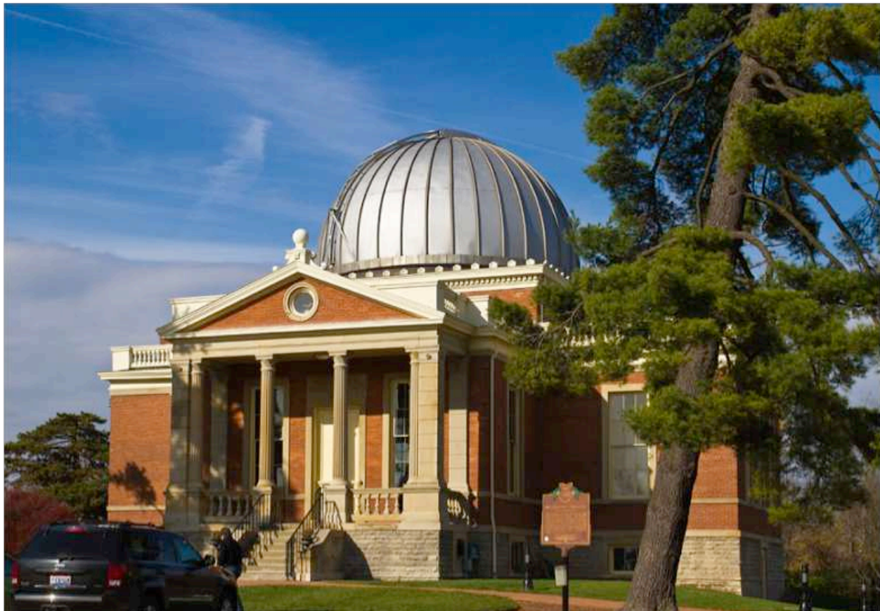
The second home of the observatory, dedicated in 1873, originally housed the 11-inch Merz and Mahler refractor. The dome is a relatively recent replacement of the brick turret with which the building was first constructed. Photos by the author.
