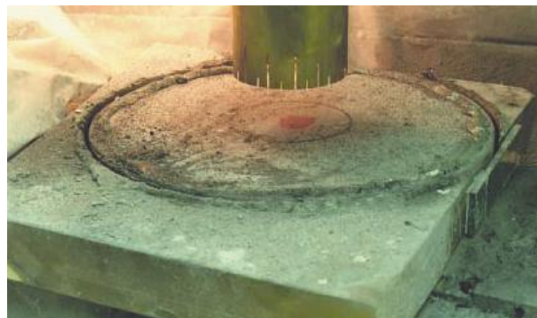
Cut the inside diameter.
