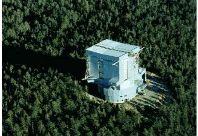
LBT construction photo used with permission
